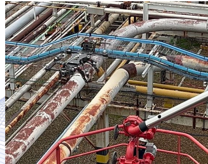
Fig. 2: Drone inspection on insulated pipes [2].
