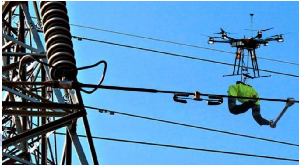
Fig. 1: Drone inspection on powerlines [1].
